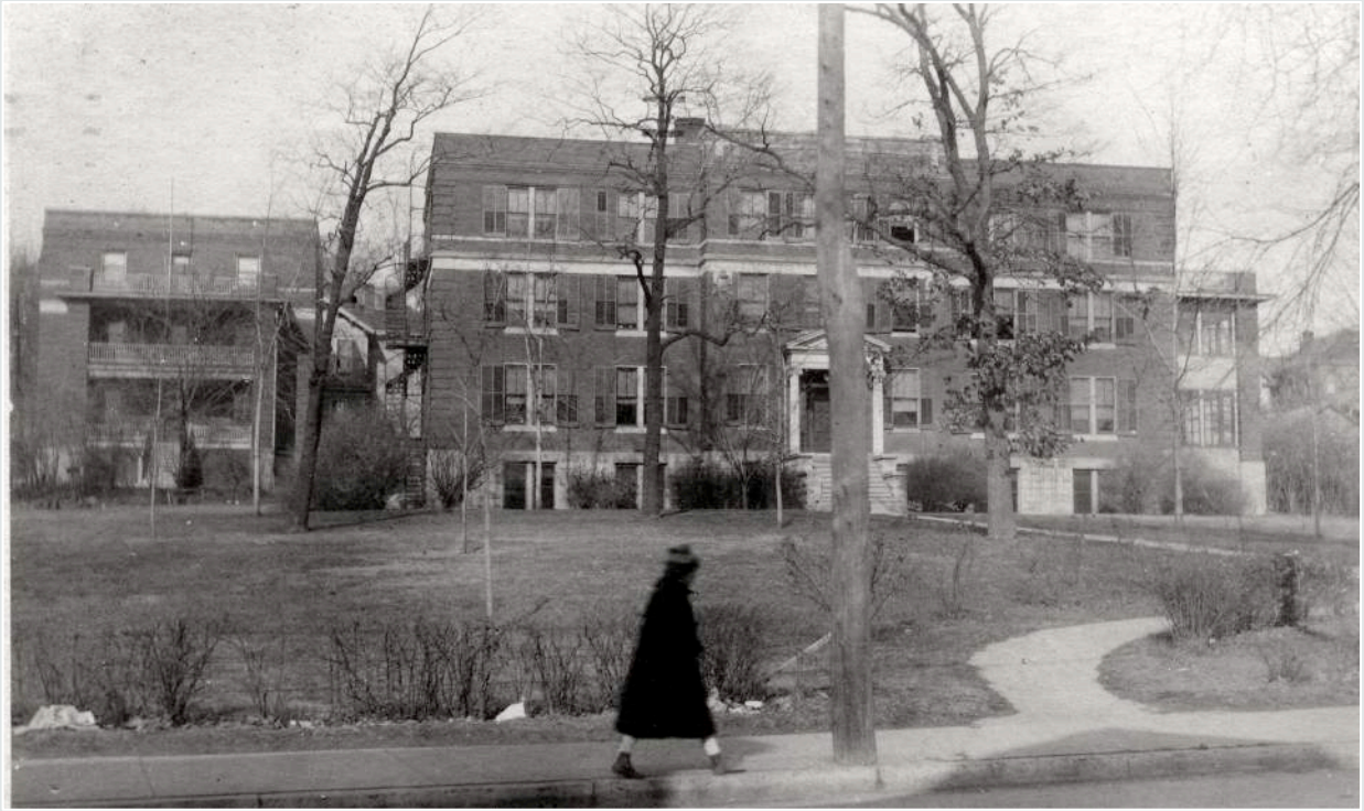
The building at right is Levering Hospital, named after A.R. Levering, co-founder of Farmers & Merchants Bank, who donated the funds to build this Hannibal health care facility. At left is the nurses' residence, which Levering also funded. STEVE CHOU COLLECTION
